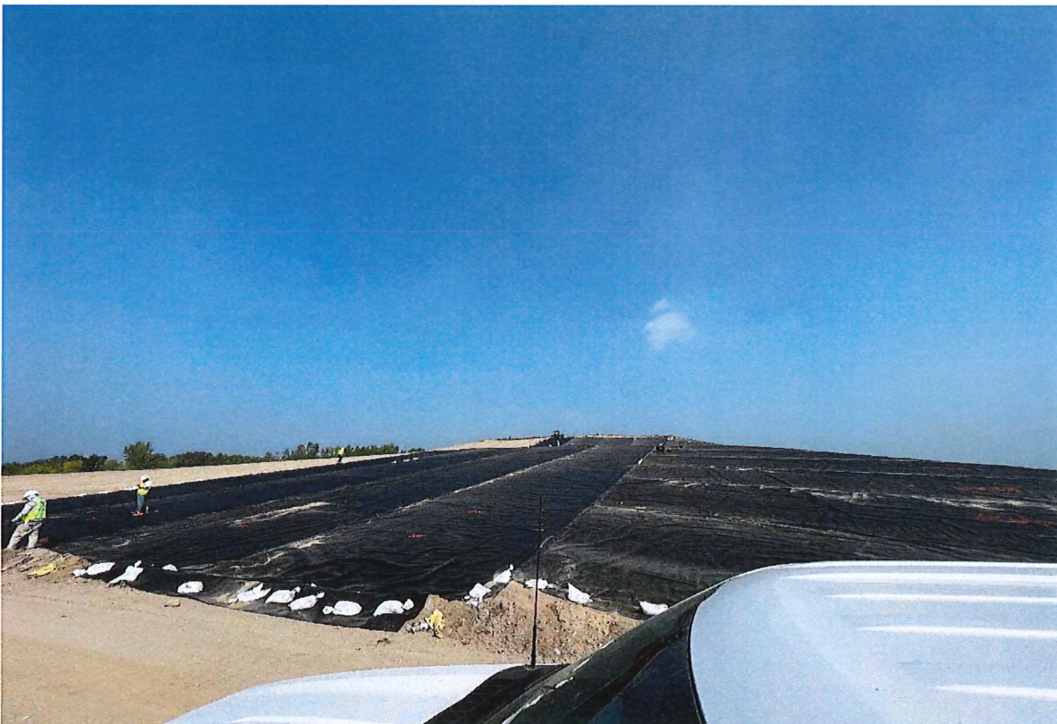
Photo 6 LLDPE geomembrane liner deployment starting on west slope; looking east. 8/30/2023
