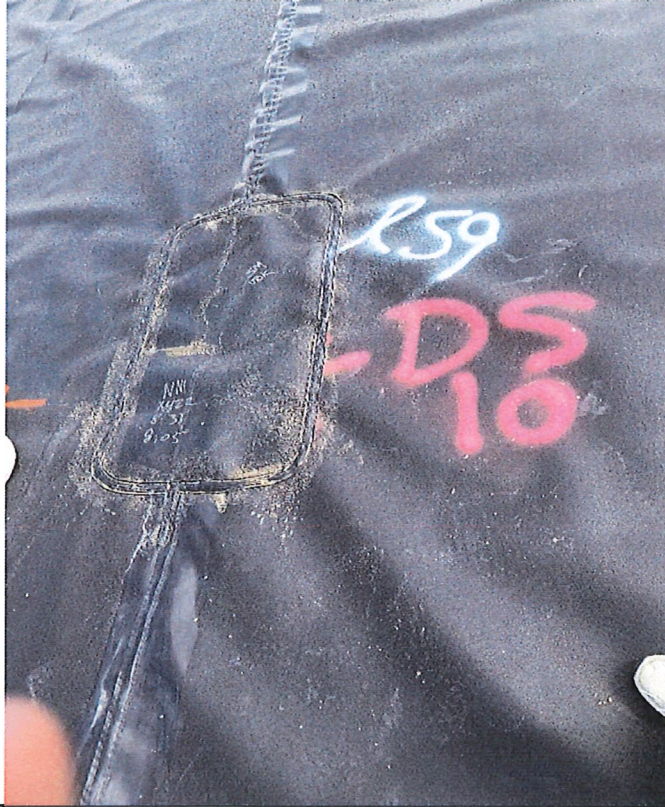
Photo 9 Vacuum tested repair of destruct sample location 8/31/2023
