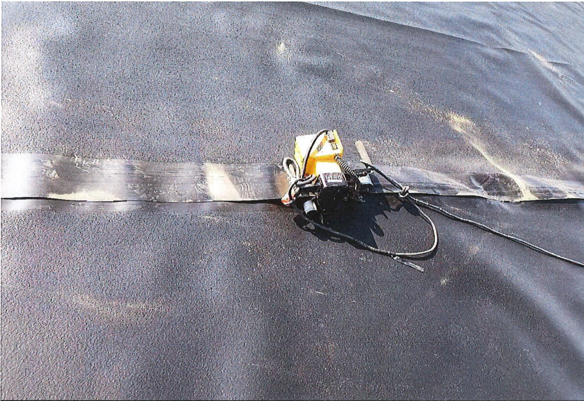
Photo 5 Dual-wedge welding of geomembrane panels 8/29/2023
