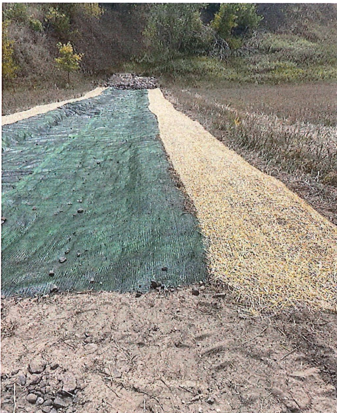
Photo 16 Turf mat placed through south stormwater channel below landfill, rip rap plunge pool at base; looking south. 9/25/2023
