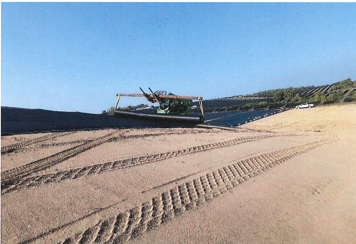
Photo 4 Skid-steer deploying geomembrane over smooth rolled buffer soil. 8/29/2023
