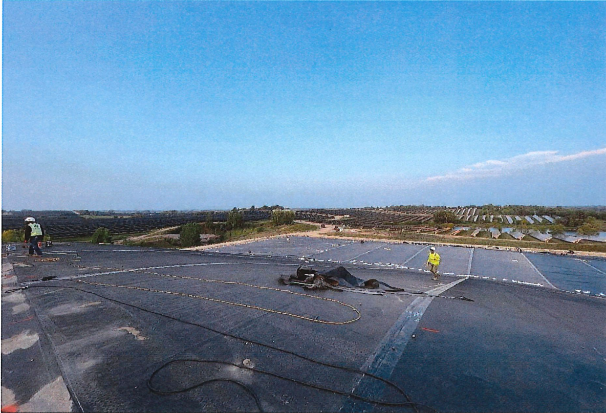
Photo 7 Geomembrane installed over final cover and tie-in; looking southwest. 8/31/2023
