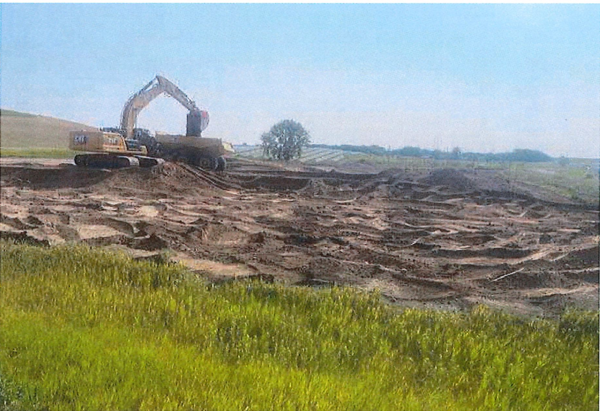
Photo 2 Common fill and buffer excavation from the borrow area; looking southwest. 7/10/2023
