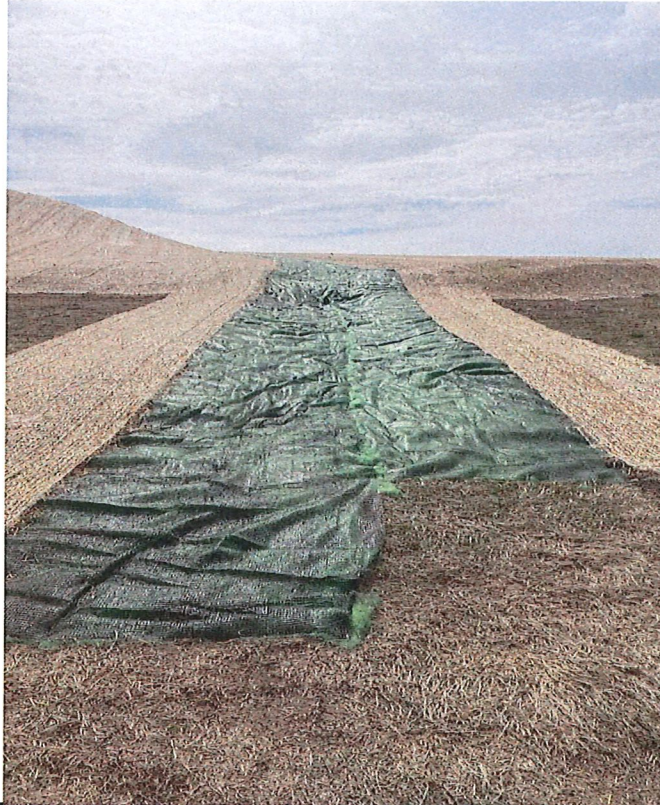
Photo 15 Turf mat placed through north stormwater channel; looking south. 9/25/2023
