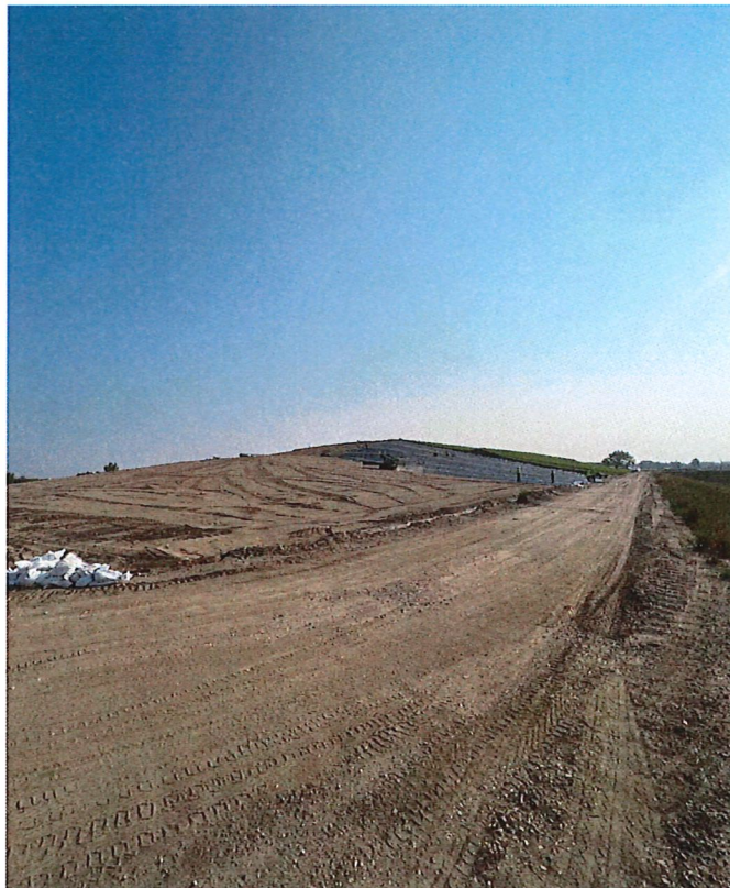
Photo 12 Granular drainage material placement over geomembrane on south slope; 9/5/2023 looking northeast.
