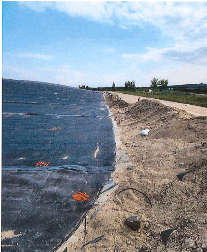
Photo 10 Extrusion welded final cover geomembrane to base liner geomembrane. 8/31/2023
