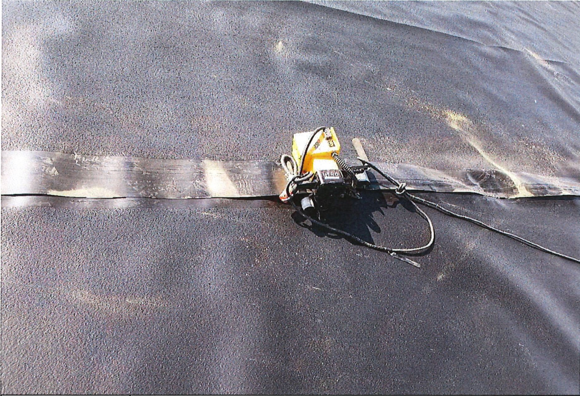
Photo 5 Dual-wedge welding of geomembrane panels 8/29/2023
