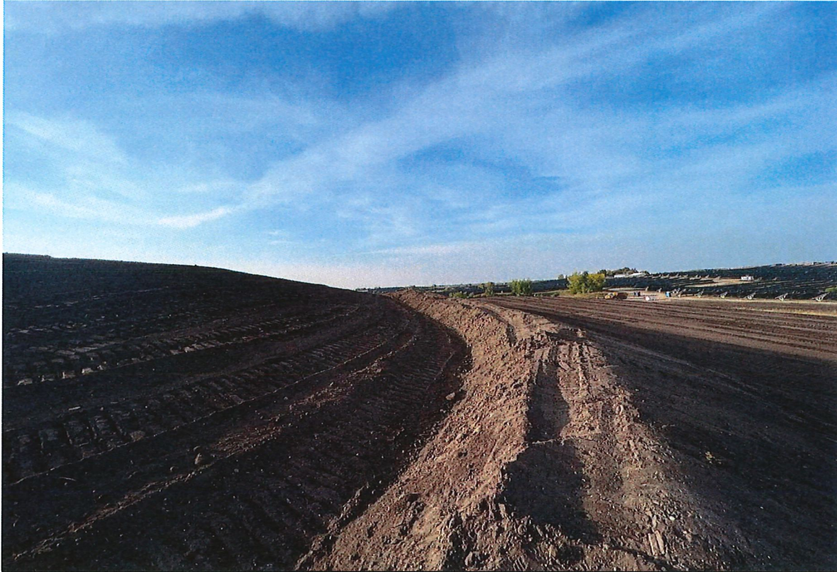
Photo 13 Topsoil rough graded on stormwater berm; looking southwest 9/20/2023
