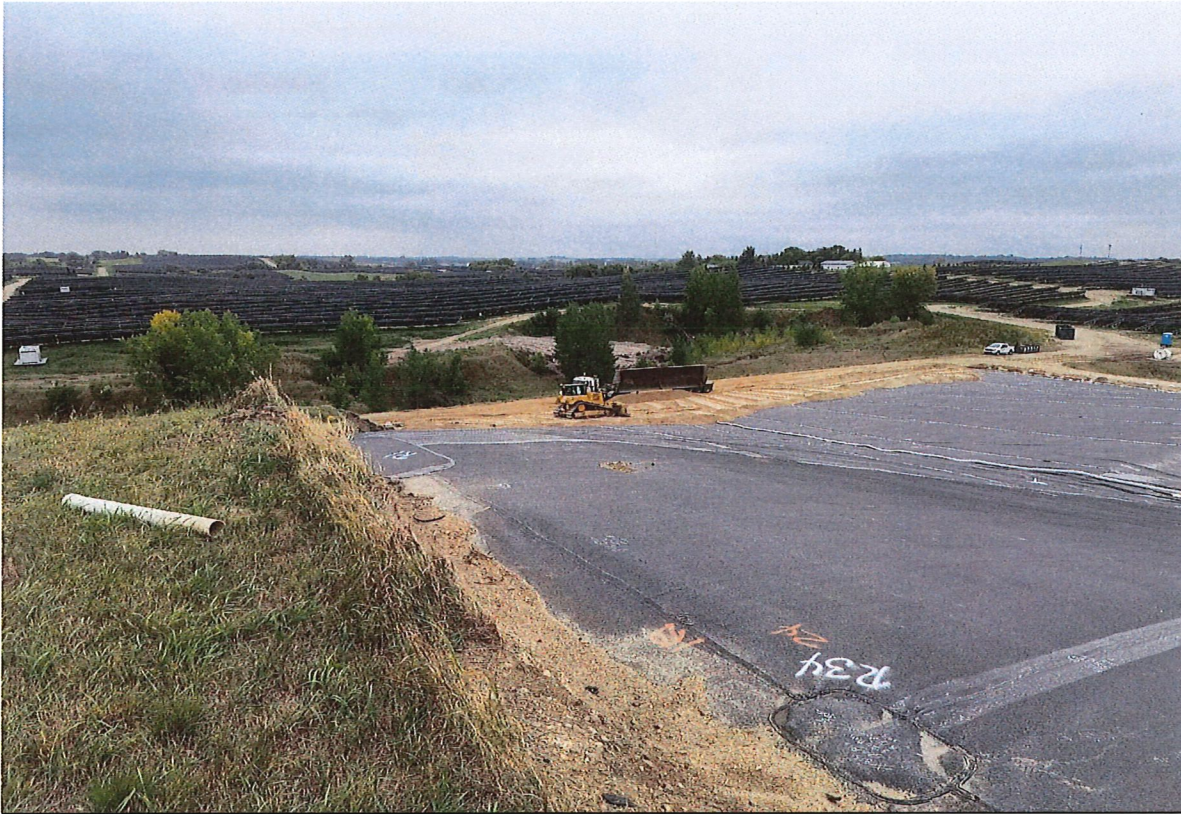
Photo 11 Granular drainage material placement over geomembrane on south slope; 9/5/2023 looking southwest.
