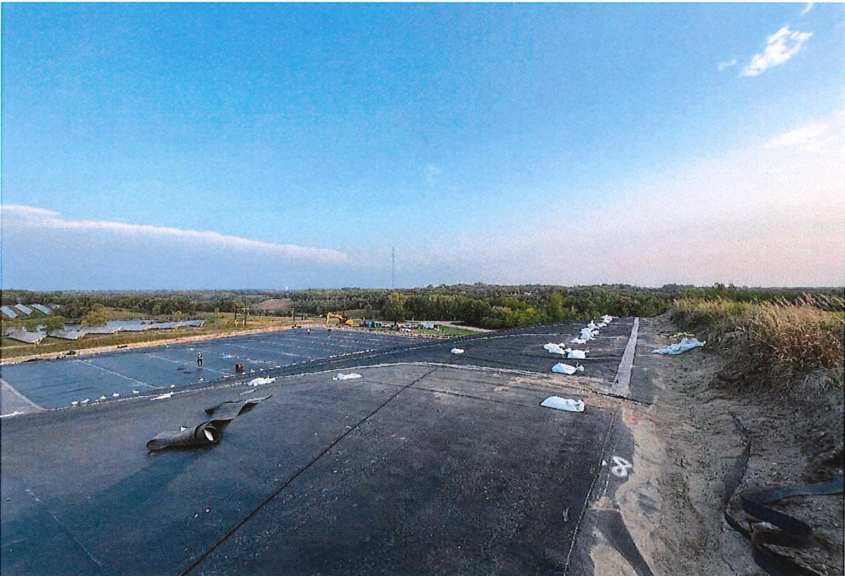
Photo 8 Geomembrane installed over final cover and tie-in; looking northwest. 8/31/2023
