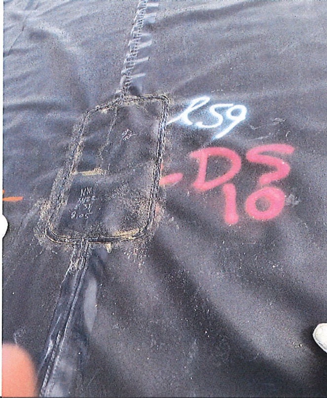
Photo 9 Vacuum tested repair of destruct sample location 8/31/2023
