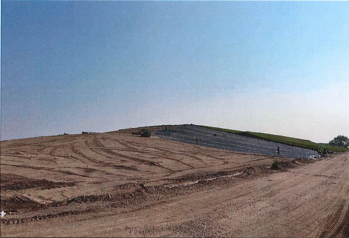
Photo 3 LLDPE geomembrane liner deployment starting on south slope; looking east. 8/29/2023
